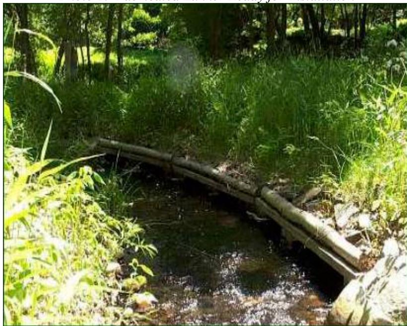
*Photo 2. Installed lunker*
