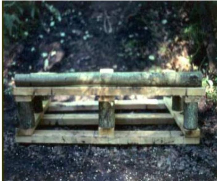
*Photo 1. Fabricated Lunker Ready for Installation*
